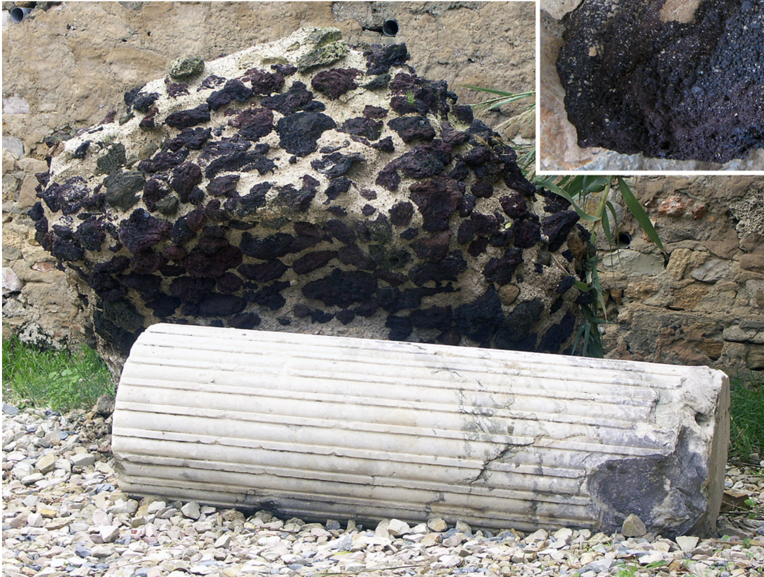
Web Figure 4 (=Figure 10A). Antonine Baths at Carthage (146-162 CE). Chunk of fallen vaulting with caementa of dark volcanic scoria imported from Sardinia. Upper right: Detail of scoria.
