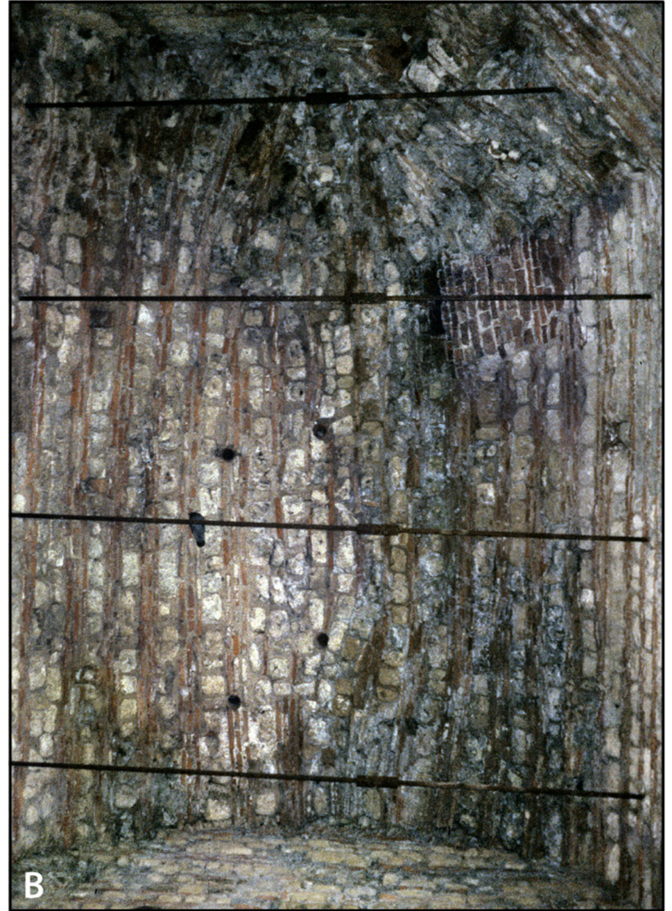
Web Figure 6 (=Figure 13). Examples of radially laid caementa combined with courses of radially laid brick. A: Substructures of the Palace of Diocletian at Split, Croatia (c. 305 CE). B: Praefurnium for caldarium of the Imperial Thermae at Trier, Germany (early fourth century CE). Note vertical tubes in vault for ventilation. The iron tie bars are modern.
