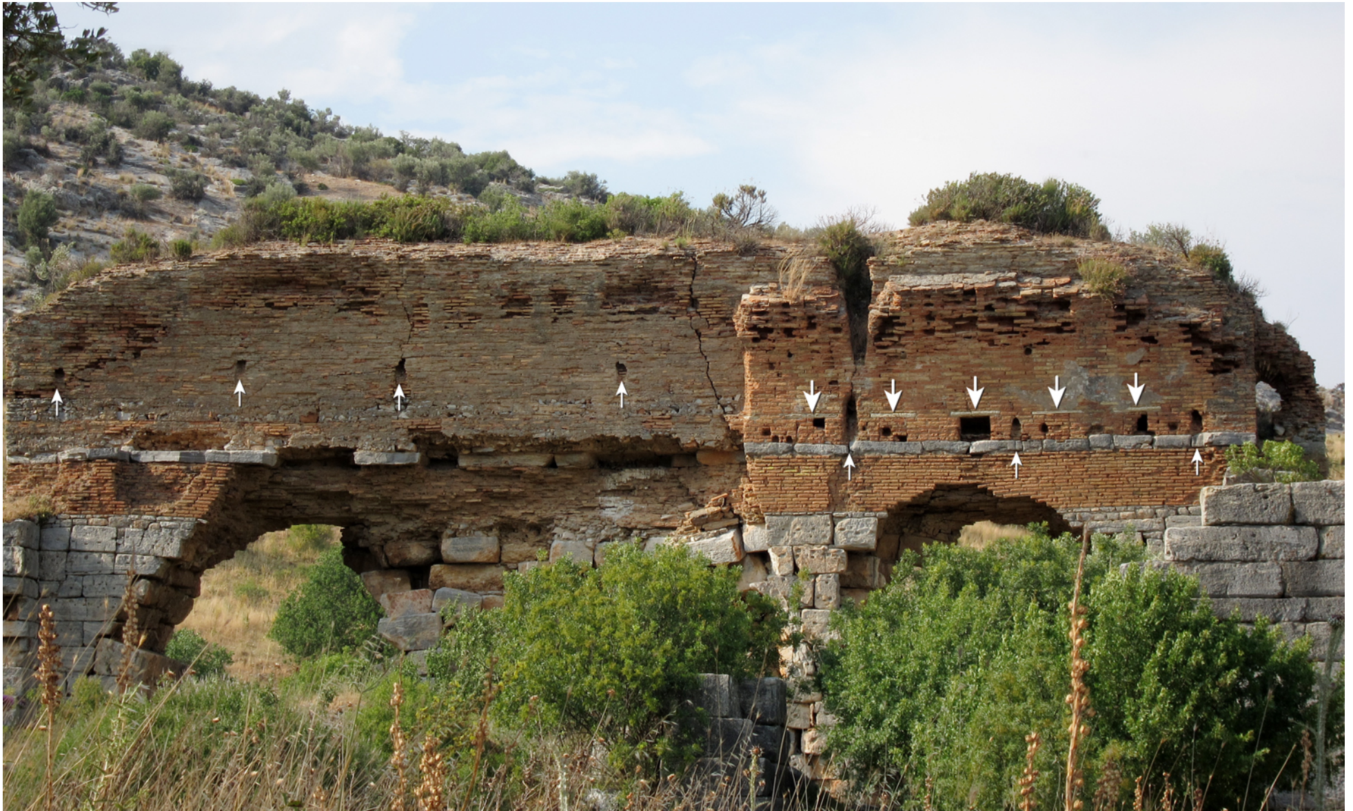
Web Figure 9. East Baths at Ephesus, Turkey (compare Figure 23A). Remains of the caldarium vault. Right side shows preserved remains of intrados of the barrel vault with the beam holes (large downward arrows), only one of which is not infilled with brick). The small upwards arrows indicate the locations of the vertical exhaust flues. Left side shows the second ring of brick where the intrados layer has fallen away.
