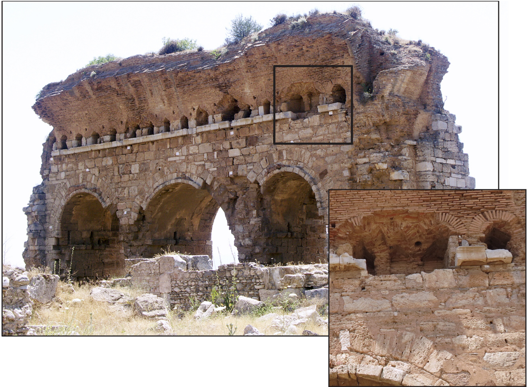
Web Figure 10. Uç Goz Baths at Tralles, Turkey (compare Figure 23B). Lower right: Detail showing the damaged beam holes. Note the vertical exhaust tube between the holes and the projecting ledge running along the intrados of the arch (bottom left), which supported the tiles for the wall heating.
