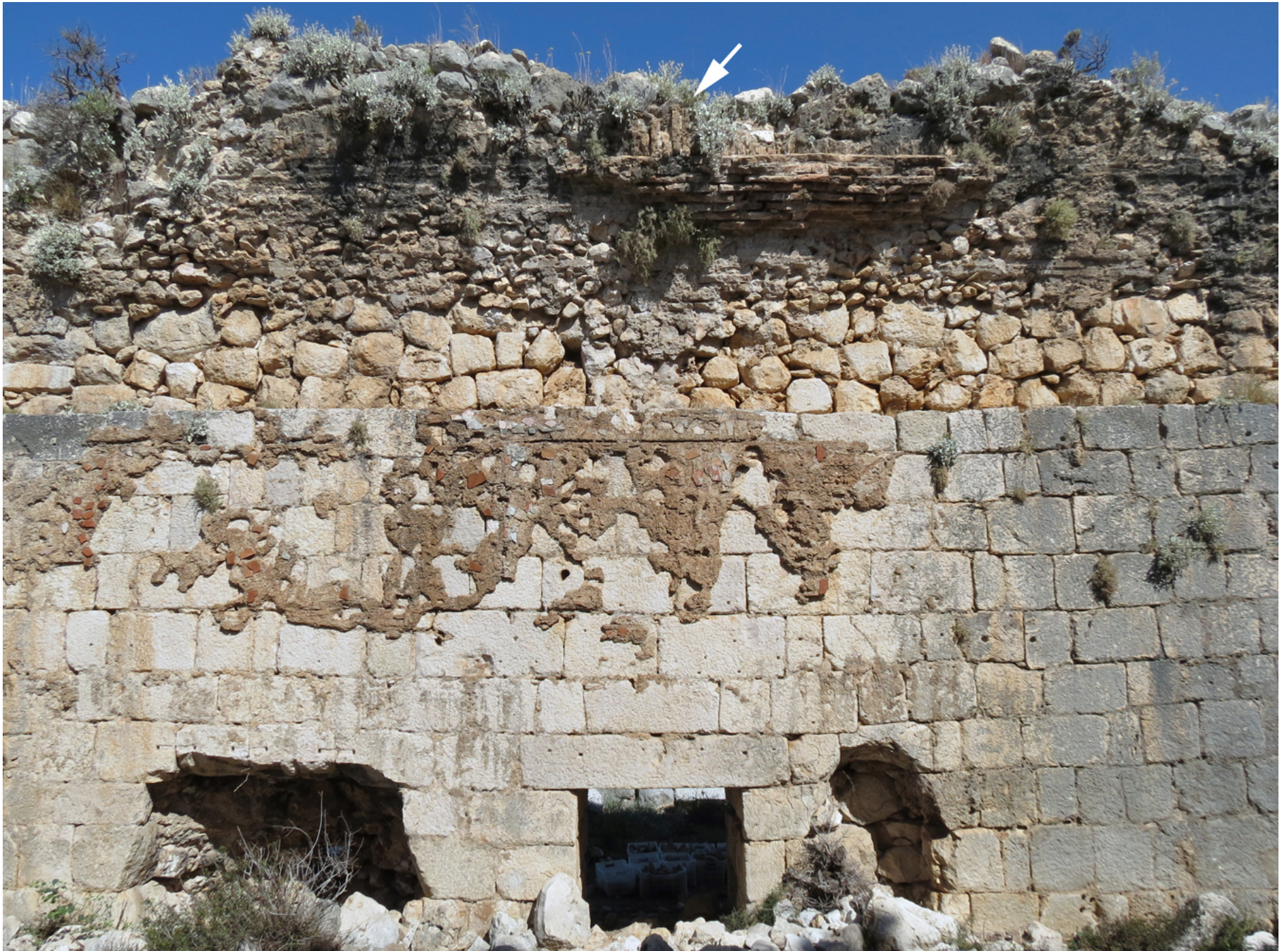
Web Figure 11. Baths of Vespasian at Patara, Turkey (mid-second century CE (?)) (compare Figure 34C). Arrow indicates remains of vertical bricks set above the radial bricks at the haunch.
