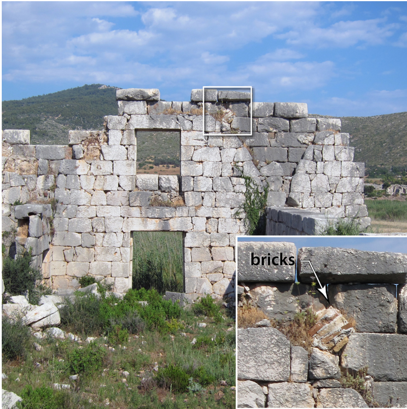
Web Figure 7 (=Figure 20). Hadrianic Horrea at Patara. Turkey (129 CE). Inset shows a few radial bricks that remain in the grooves carved into the front wall.
