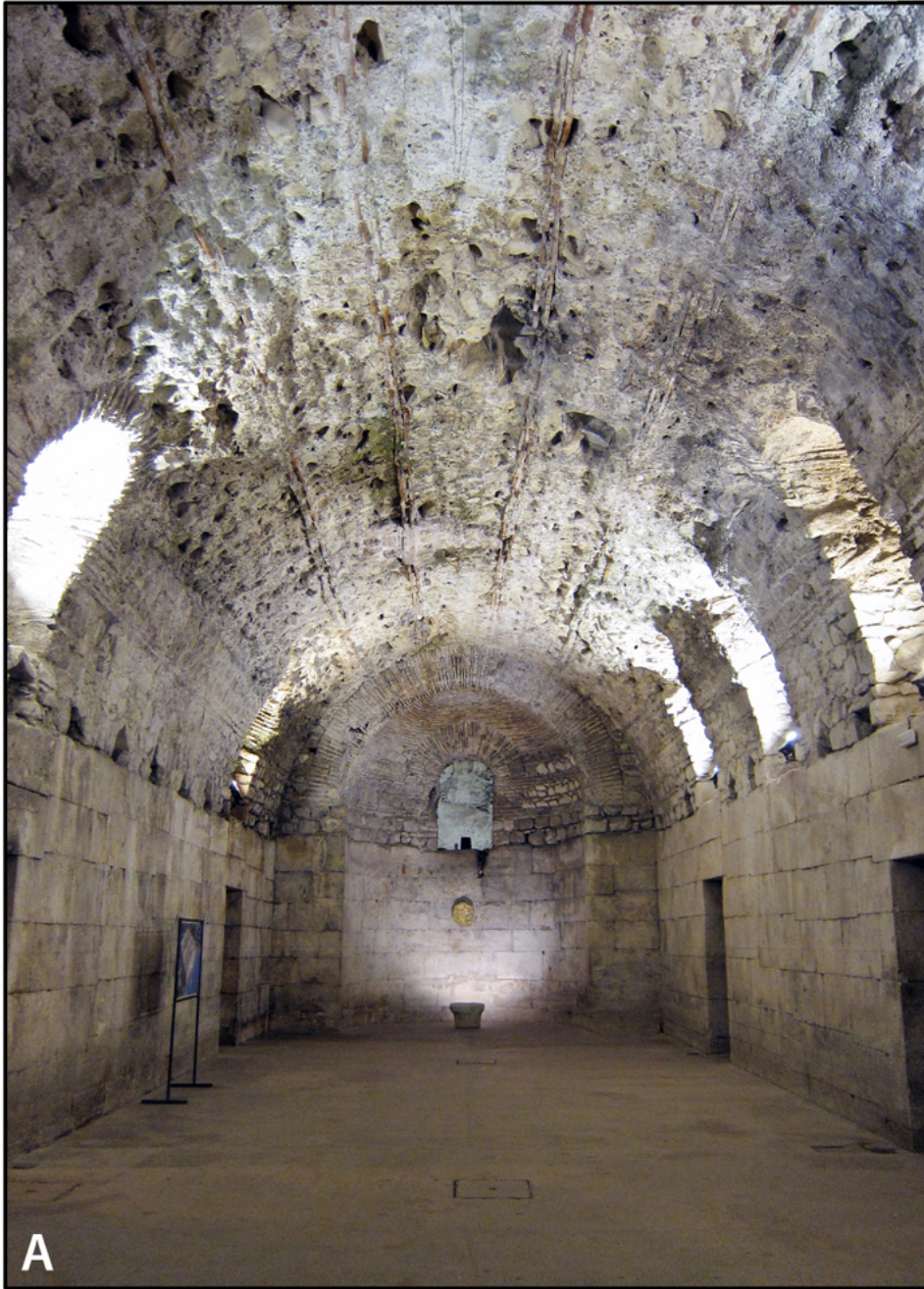
Web Figure 6 (=Figure 13). Examples of radially laid caementa combined with courses of radially laid brick. A: Substructures of the Palace of Diocletian at Split, Croatia (c. 305 CE). B: Praefurnium for caldarium of the Imperial Thermae at Trier, Germany (early fourth century CE). Note vertical tubes in vault for ventilation. The iron tie bars are modern.
