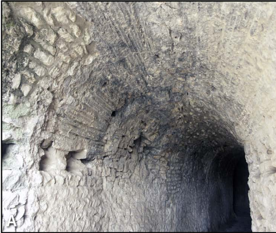
Web Figure 26 (=Figure 78). "Licinian" Baths at Dougga, Tunisia (third century CE). Two substructure galleries built using different techniques. A. Vault with impressions of reed mats along intrados. Centering holes visible at left. B: Vault with remains of vaulting tubes along intrados visible at left (Photo: Miles Lewis).
